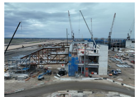
WSI terminal construction
