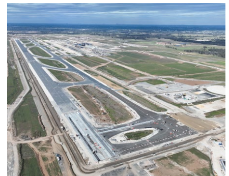
WSI runway construction
