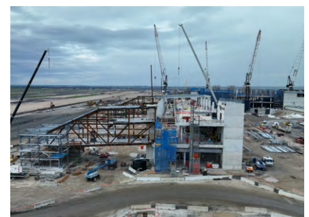
WSI terminal construction
