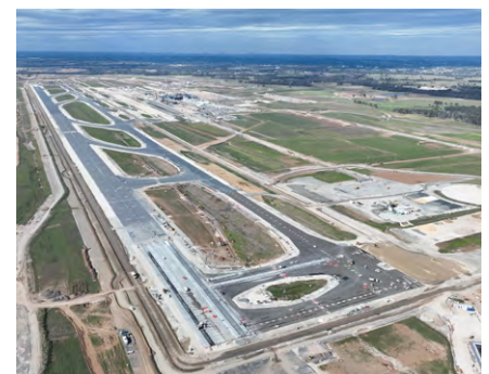
WSI runway construction
